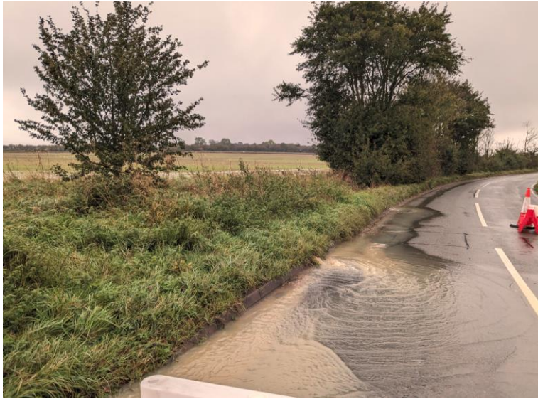
Figure 11: Field northeast of site showing flooding onto Yarnton Road caused by surcharging culvert and highway drainage
